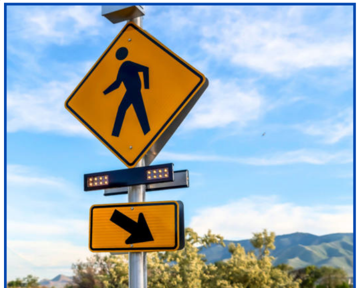
Rectangular Rapid Flashing Beacon
