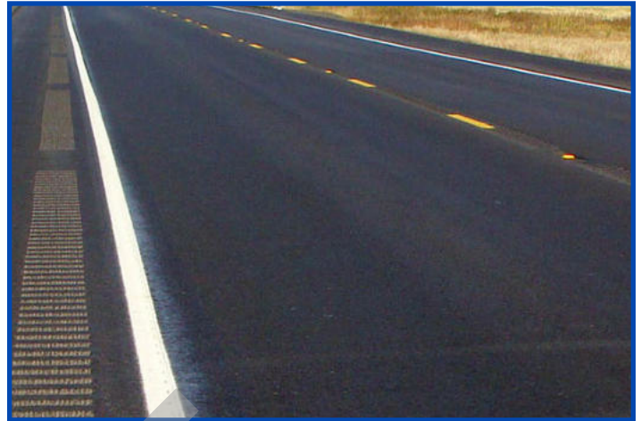
Shoulder rumble strips and centerline rumble strips. Source: FHWA
