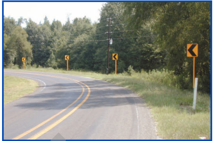
Chevron signs with retroreflective strips on sign posts installed along a curve. Source: FHWA
